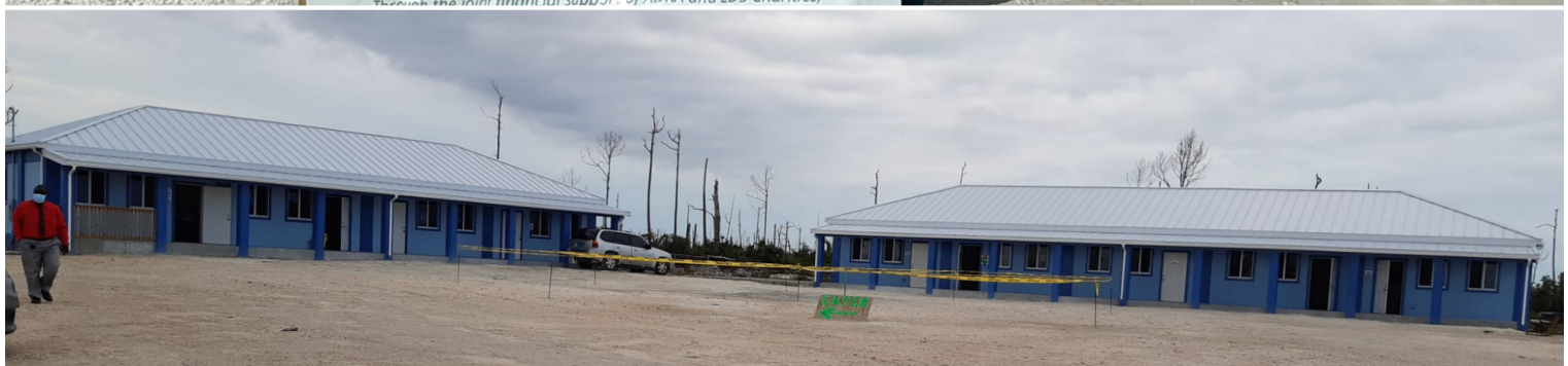
Little Darlings, Abaco (cover photo- completed school campus)
